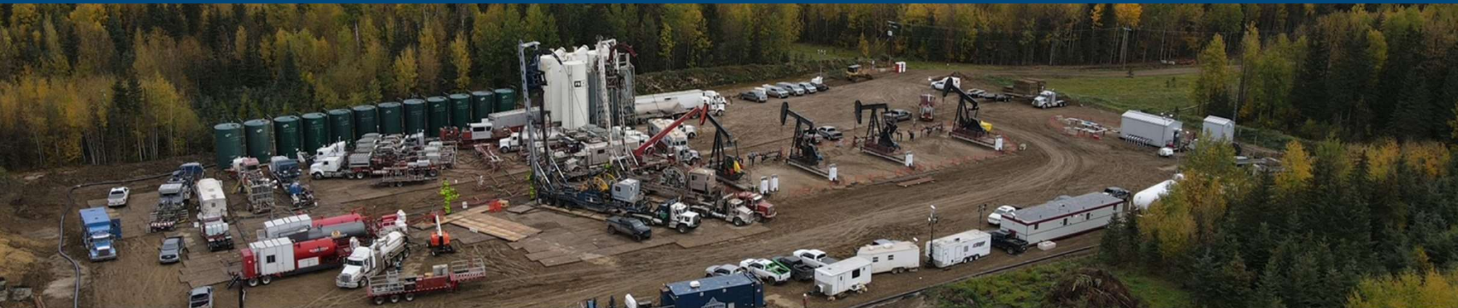
Fracture completion operations at InPlay 7 well pad in Pembina Region (October 2025)
