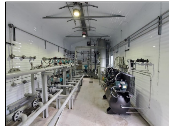
Sites have been converted to instrument air to reduce venting and fuel gas
